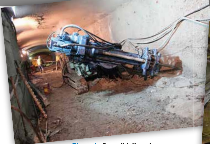
Phase 1 Consolidation of the zone between the tubes
